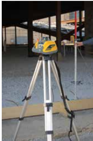
Exterior application setting forms
